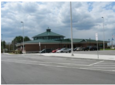
Turnpike Visitor Center
